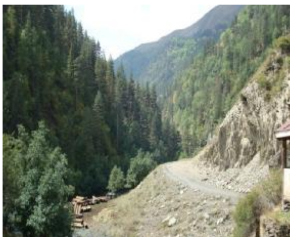
Hydro power facility construction site
